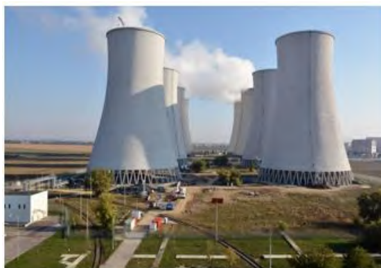
Before demolition of 4 cooling towers (09/2017)
