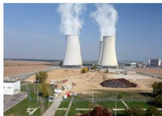
After demolition of 4 cooling towers (10/2018)
