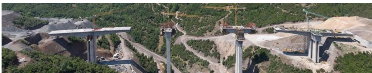
Bridge B3 during construction
